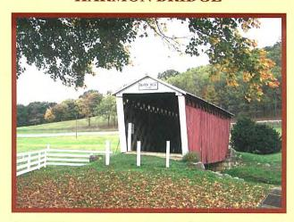
Harmon Bridge and Trusal Bridge are companion bridges located on the South Branch of Plum Creek just off Five Points Road. Both the Harmon and Trusal bridges are constructed with town lattice trusses. The bridges are located in a very picturesque farm setting.
